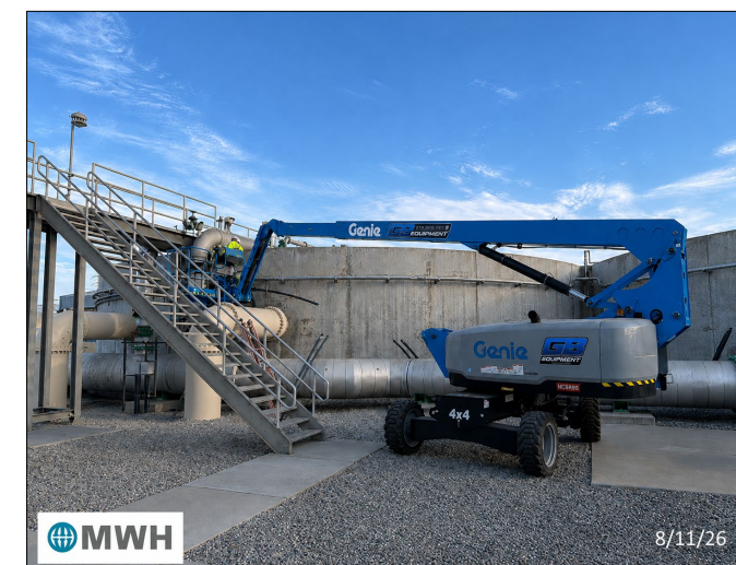
Electrical subcontractor installing PVC coated conduit on south side of aeration basin
