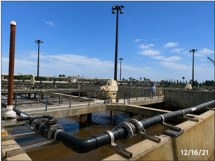
RP-1 Existing Aeration Basins
