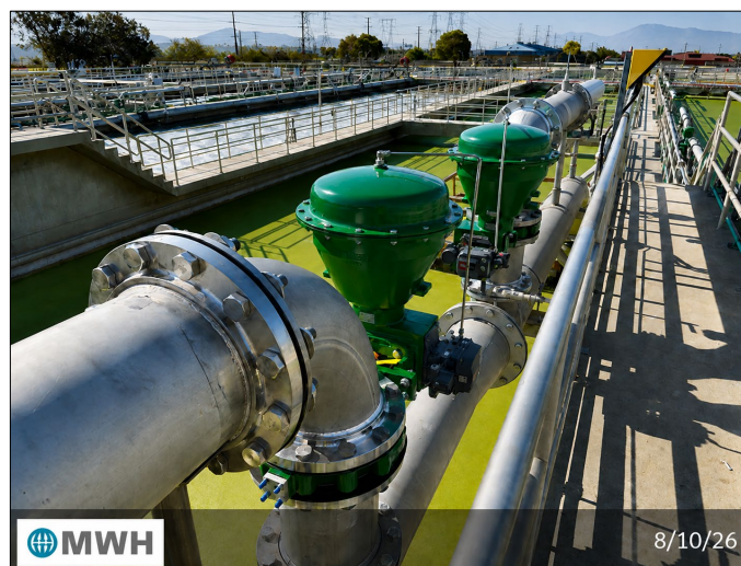
10-inch pneumatic valves installed on Aeration Basin trains 1 & 2
