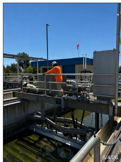
Tertiary Filter Rehabilitation
