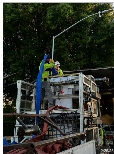
CIPP Liner Installation
