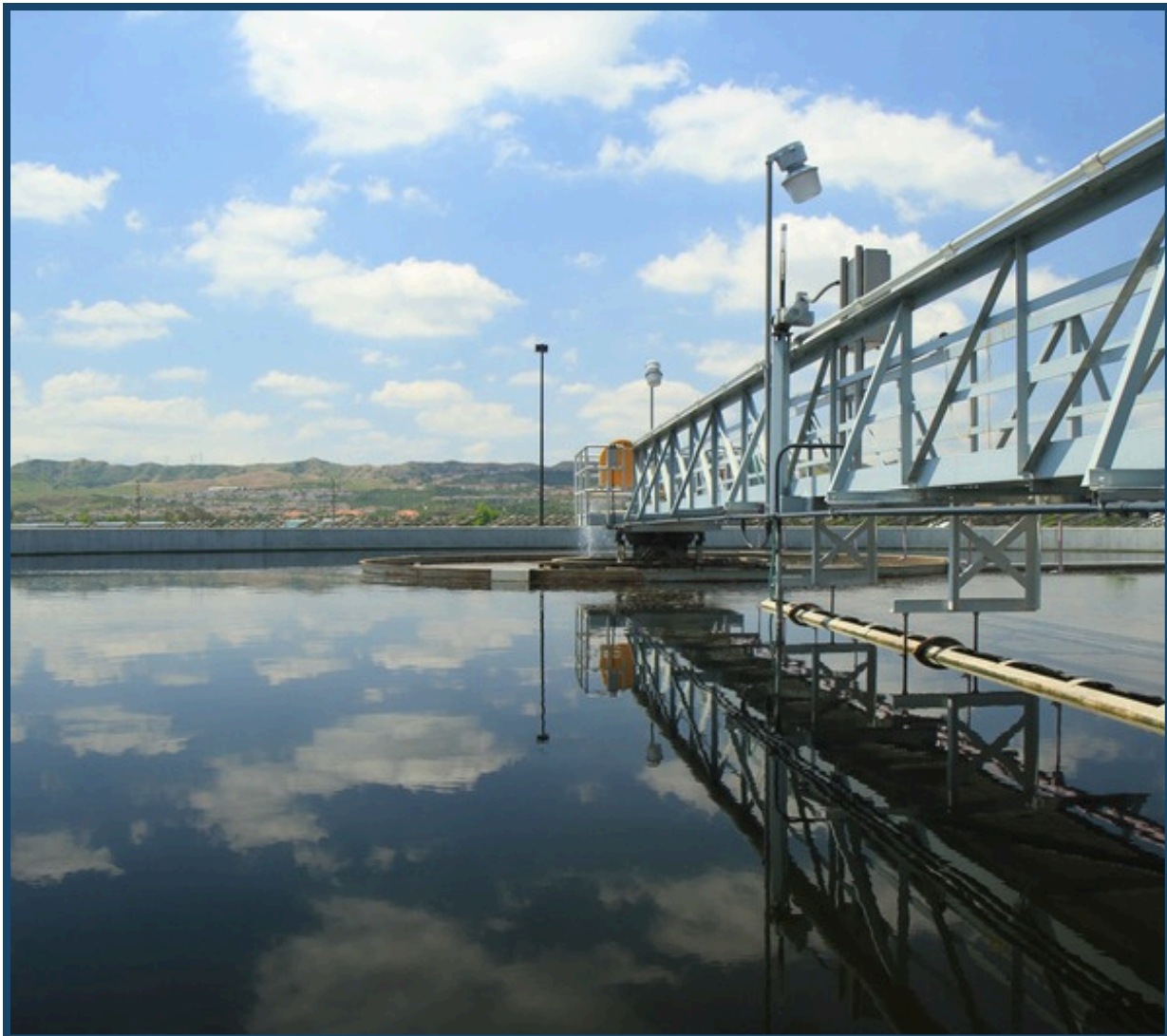
Regional Water Recycling Plant No. 5 (RP-5) in Chino, CA has the current capacity to treat 16.3 million gallons of wastewater per day, equivalent to just under 25 Olympic-sized swimming pools.
