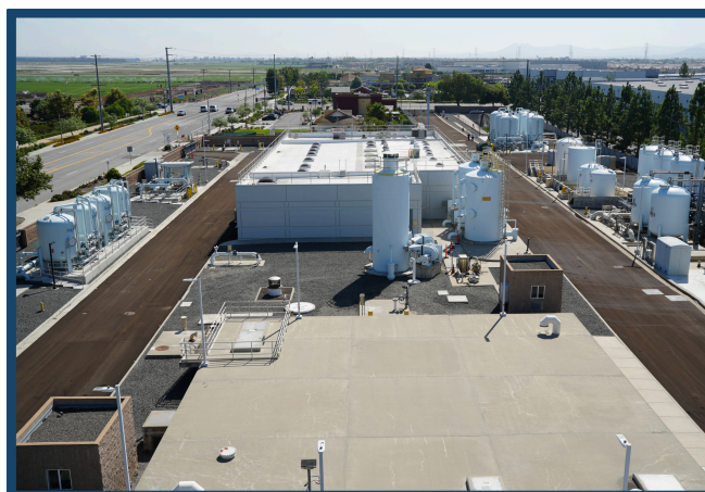
The Chino Desalter I processes 14 Million Gallons per Day of groundwater from the Chino Basin using Reverse Osmosis and Ion Exchange for the removal of nitrate and total dissolved solids.
