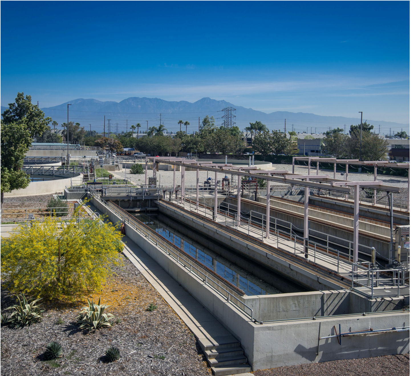
Carbon Canyon Water Recycling Facility Chino, CA - The Aerial Contact Basin allows dissolved gasses in the water to be removed.
