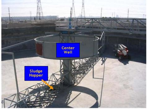
Figure 3-6: Primary Clarifier Stilling Well and Sludge Hopper
