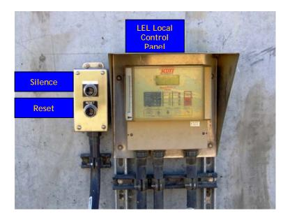
Figure 3-32: Local Display and Reset for H<sub>2</sub>S Monitor in Primary Clarifier Area
