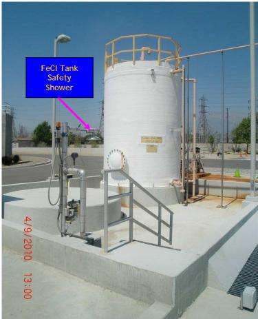
Figure 3-35: Ferric Chloride Tank Safety Shower
