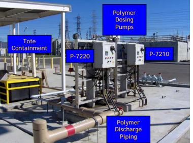
Figure 3-10: Polymer Tote Storage and Dosing Systems
