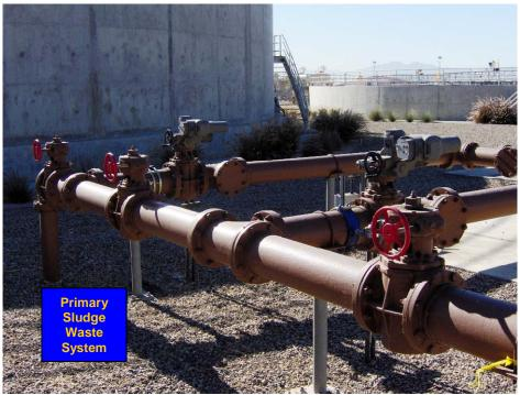
Figure 3-7: Primary Sludge Wasting System
