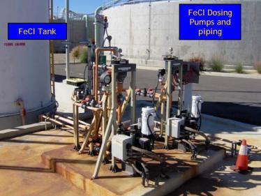
Figure 3-8: Ferric Chloride Tank and Metering Pumps
