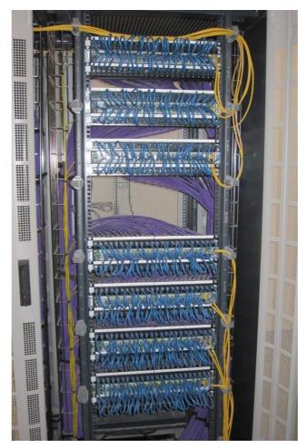
**Figure 4.** Cabinet layout after patching with 0.25m patch leads, showing groups of two 1U 24-port Cat.6A patch panels, located above and below a 48 port PoE switch. Note gaps left to facilitate maintenance and airflow. Note also the dressing of the infrastructure cables to facilitate the switch installation.
