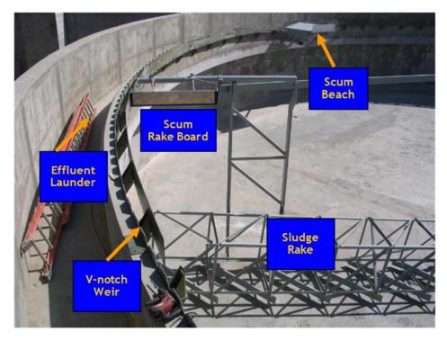
Figure 3-5: Primary Clarifier Internal Components
