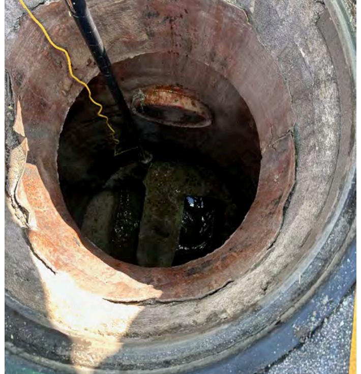
Task A (Photo A5): Inspection of Siphon manhole.
