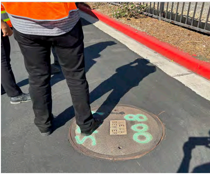
Task B (Photo B3): Lowest upstream manhole adjacent to station.
