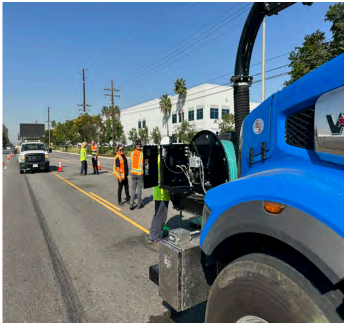
Task A (Photo A7): View west of siphon cleaning site.
