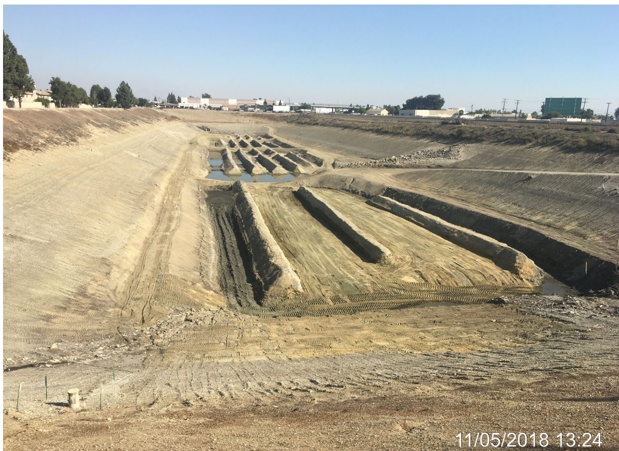
Brooks Basin – Post Floor Regrading – Two Windrows Removed to Fill Deep Stagnant Areas
