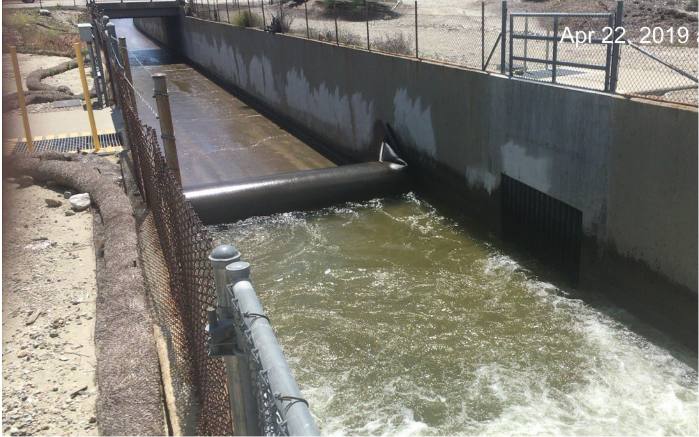
Rubber Dam used to Divert Imported Water to College Heights From San Antonio Channel
