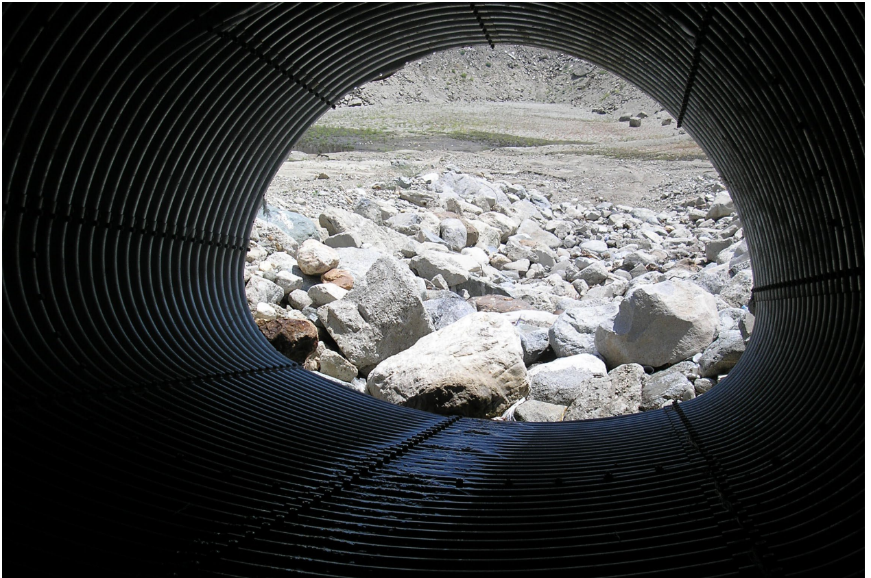
Large North-South Storm Drain From Foothill Blvd Used to Move College Heights Rubber Dam Diversions into Upland Basin
