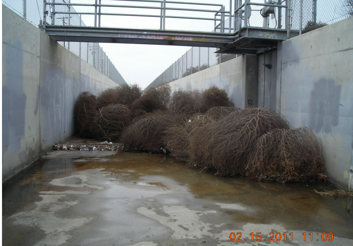
Cleaning Off State Street Storm Drain – Tumbleweeds Has Vandalism Kept This Inlet From Being Re-Automated?
