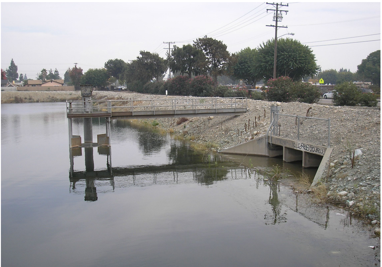
Montclair 1 – Outlets: Vertical Gated Riser and Box Culvert (November 2005)
