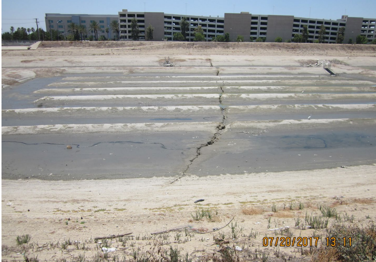
Ely 3 – Floor Crack – Before Compacted in 2019
