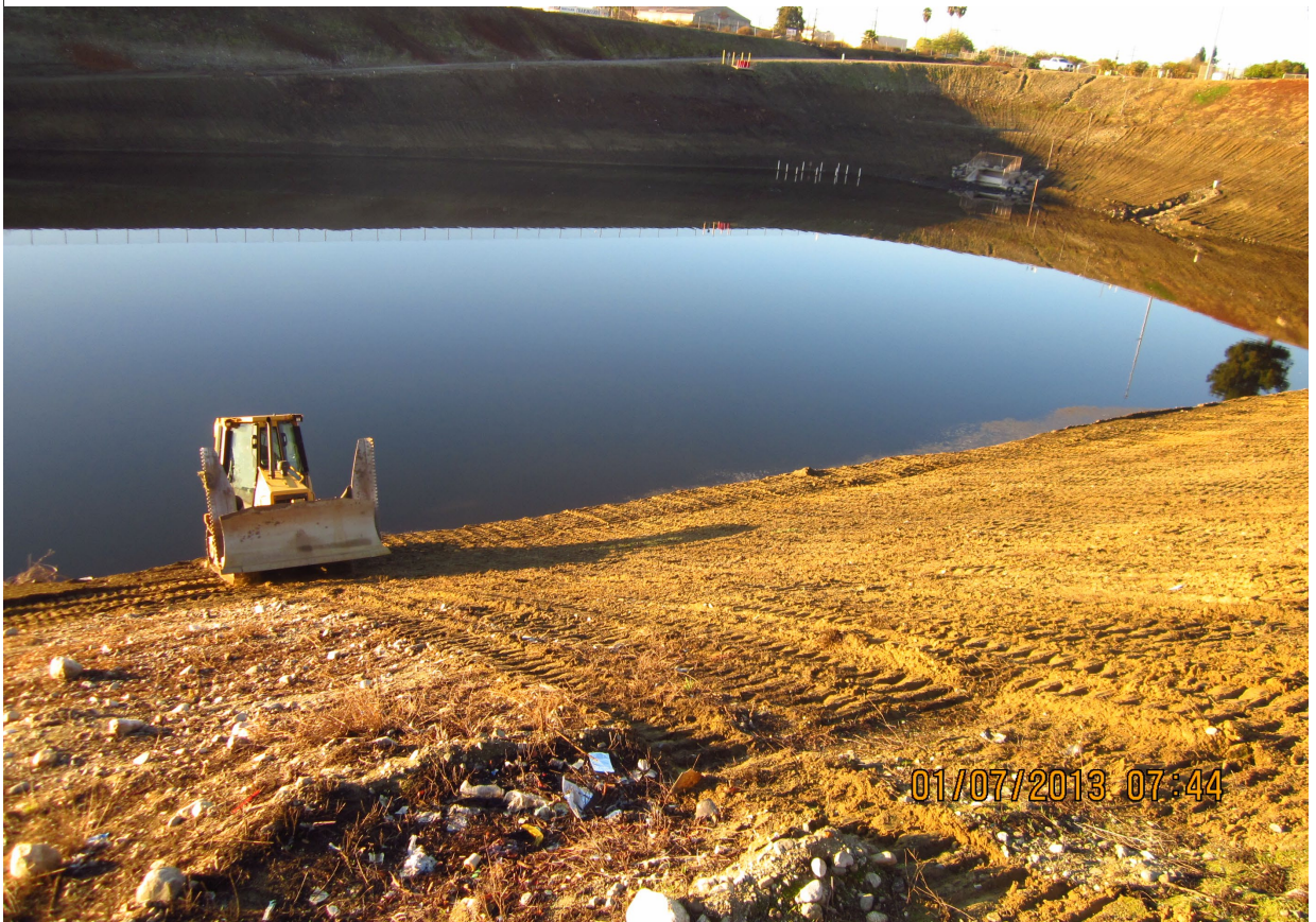
Brooks Basin – January 2013 – Restoring Slope Infiltration Does IEUA Still Sample Its Lysimeters?
