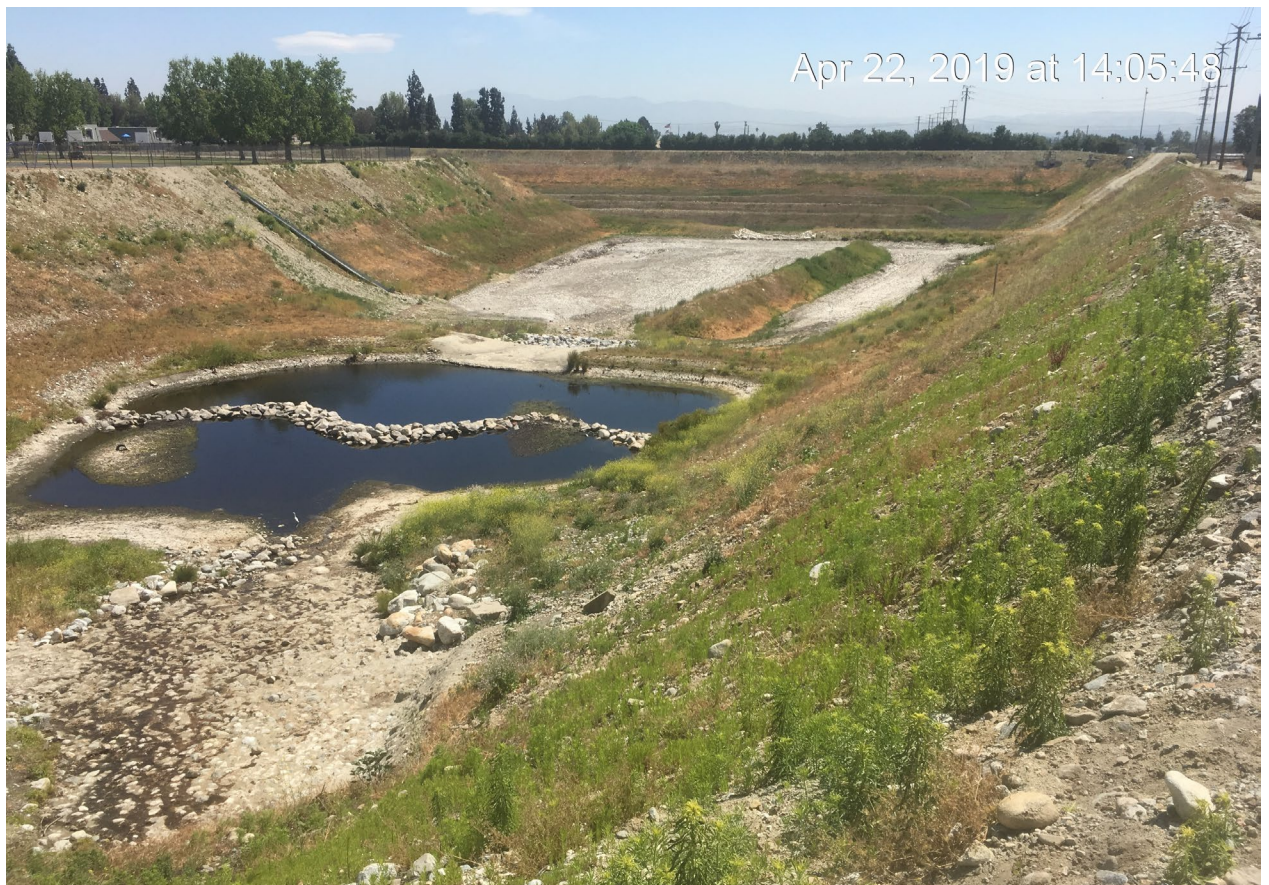
Montclair 2 – Newly Rebuilt Inlet Energy Dissipater Area – Is This Really A Wetlands?
