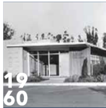
CBMWD completes the construction of 1 st headquarters in Ontario.
