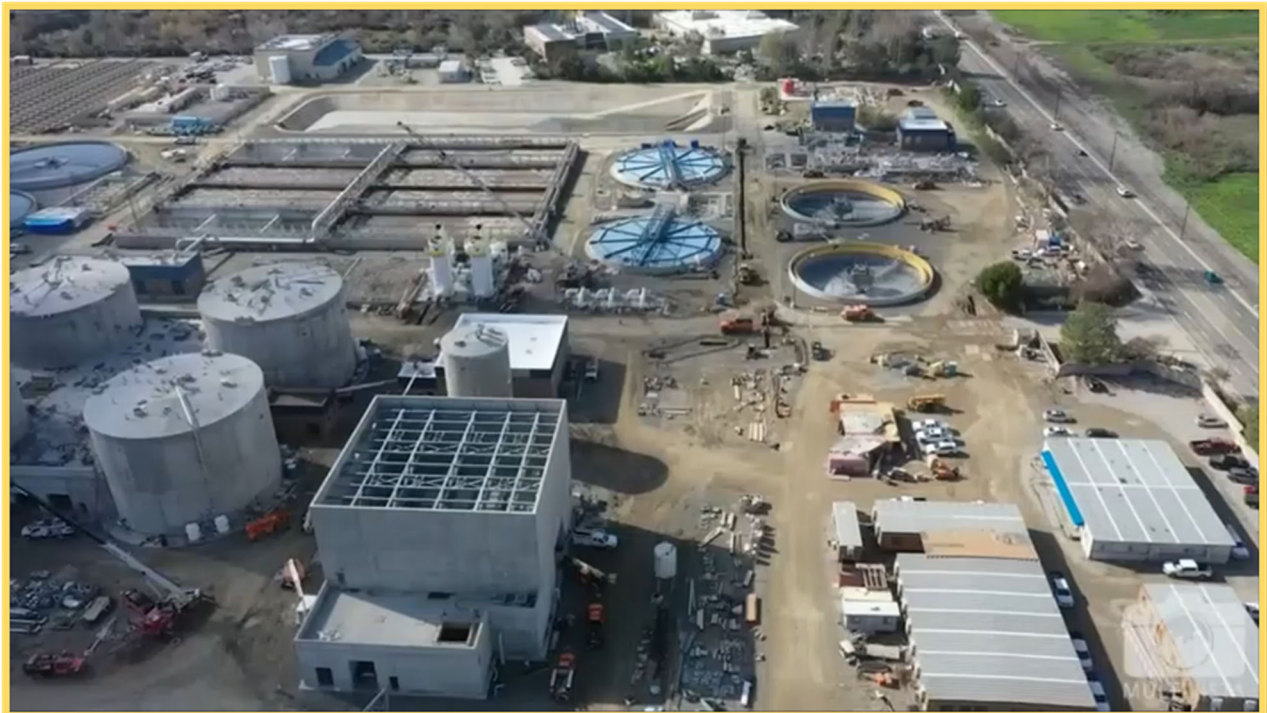
RP-5 Flyover – January 2023
