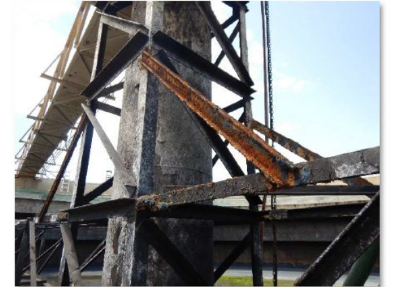
Photo 3-17. Center pier in good condition; corrosion on support angles.
