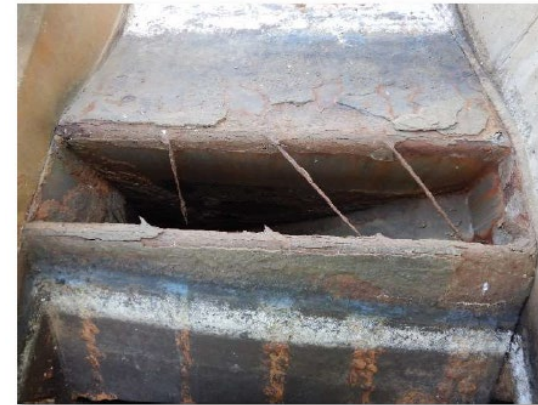
Photo 3-10. Stiffening bars of scum trough within influent channel are in VANDA Level 5 condition.
