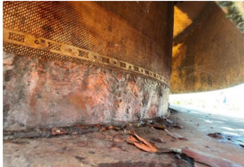
Corrosion on Center Vent Neck
