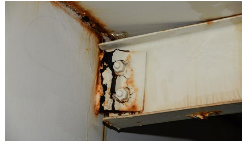
Gusset Plate to be Replaced
