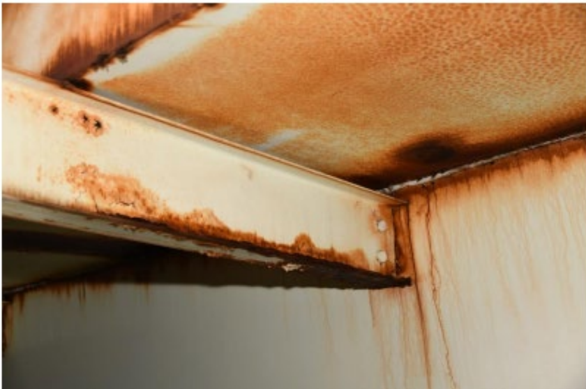
Cracked Coating Along Rafter
