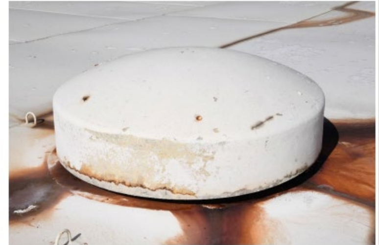
Corrosion on 4' Diameter Center Vent Cover
