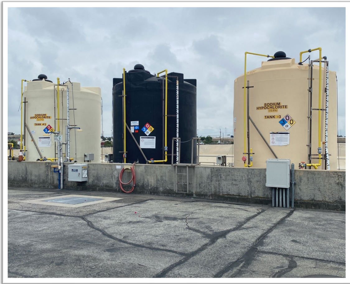
RP-1 Sodium Hypochlorite Storage Tanks
