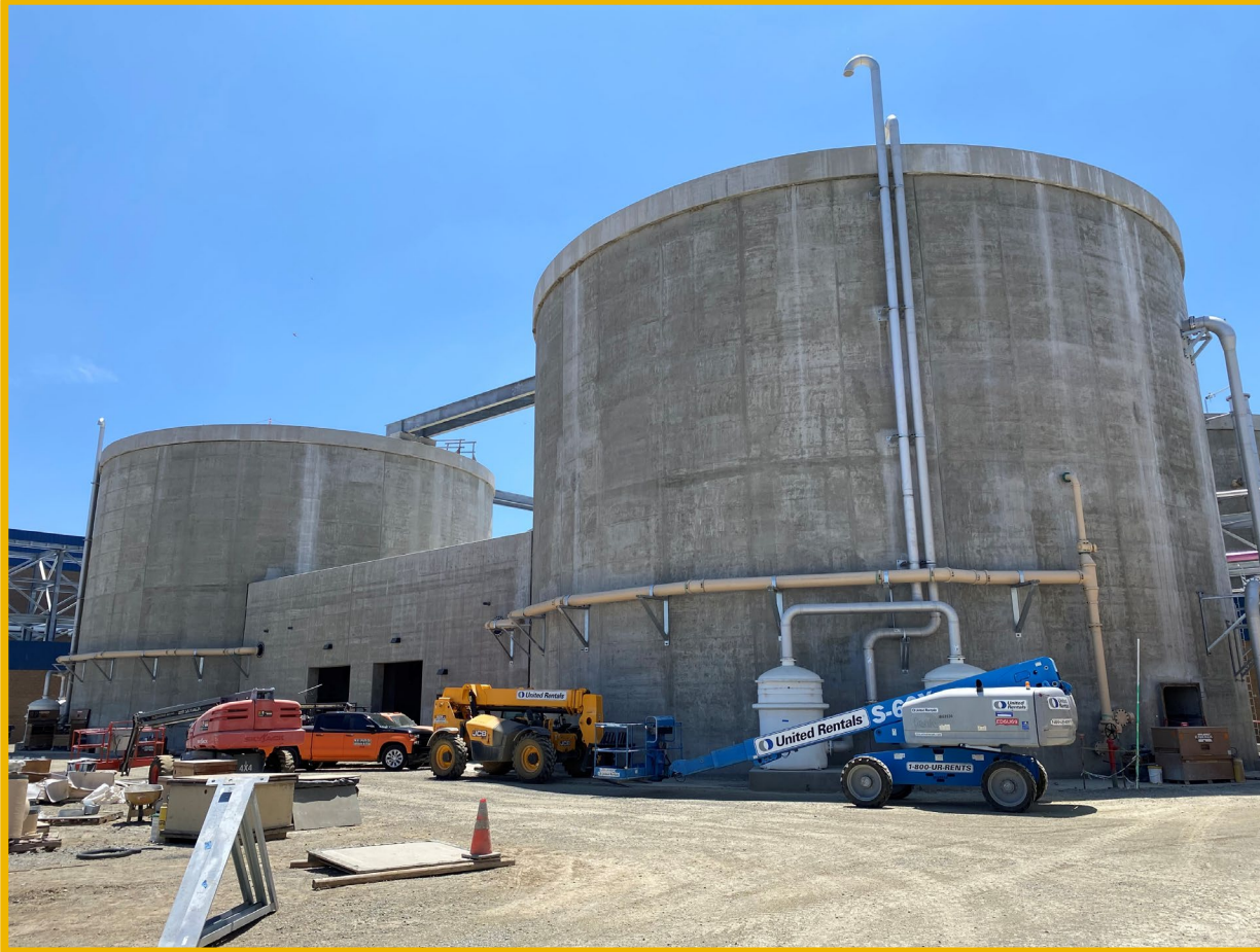
Gas Phase Digester Tank and Building
