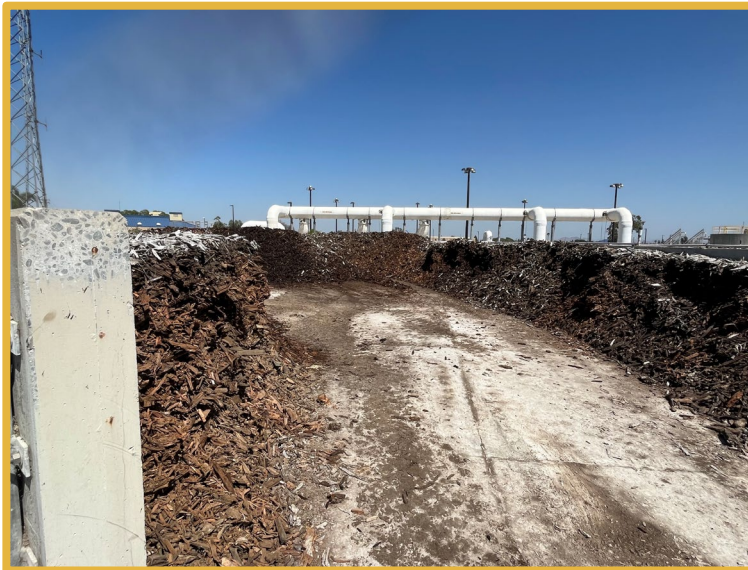
Removal of Media in Biofilter (left) and Plugged Perforated Holes (right)
