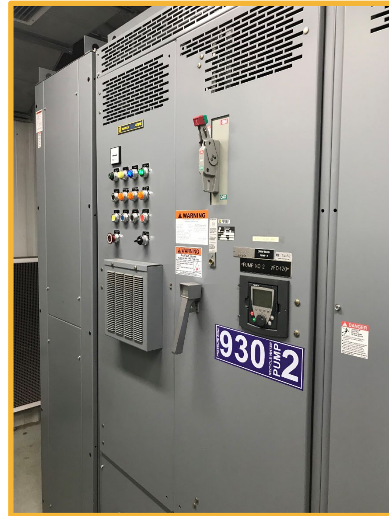
930 RW Variable Frequency Drive (VFD)
