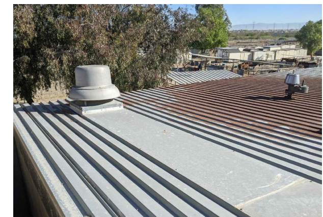
Rusted Corrugated Metal Roof
