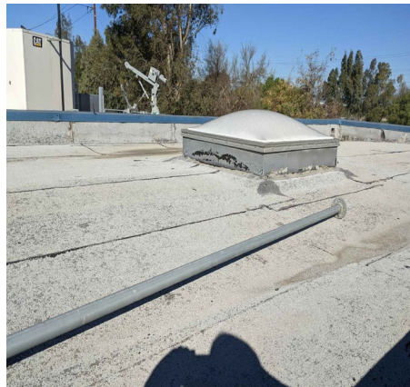
Replace Skylight Remove ACM Mastic
