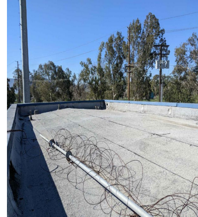
Patch/Install B.U.R Remove ACM Mastic
