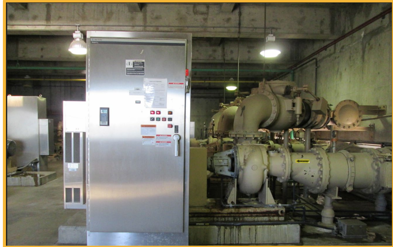
RAS Variable Frequency Drive (VFD)
