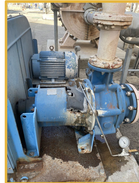
Existing Sludge Recirculation Pump
