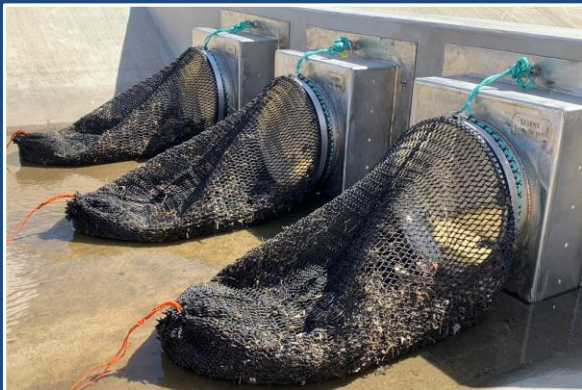
Completed Trash Nets at RP-3
