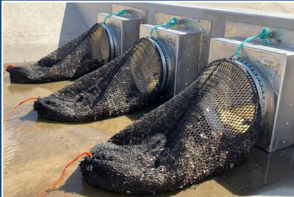
Completed Trash Nets at RP-3
