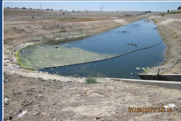
Trash Boom Tested at Jurupa Basin
