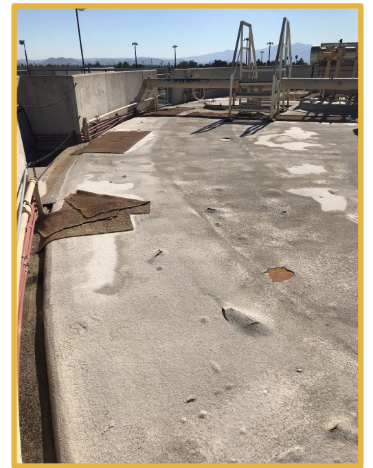
Digester 7 Roof Foam Cracks
