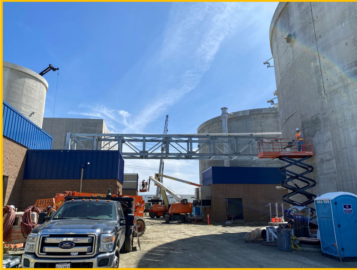
Gas Phase Digester Pipe Bridge
