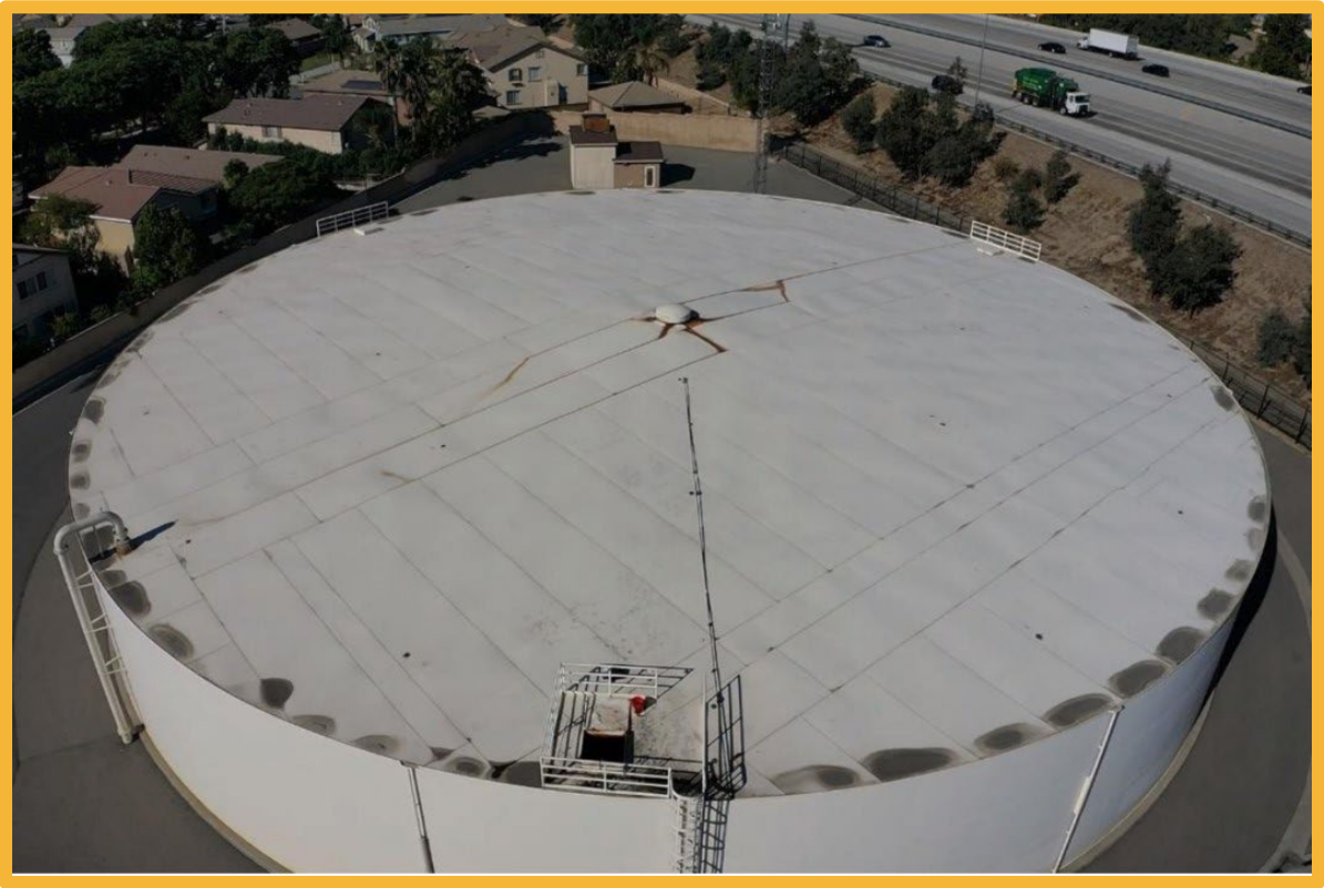
Ponding on roof
