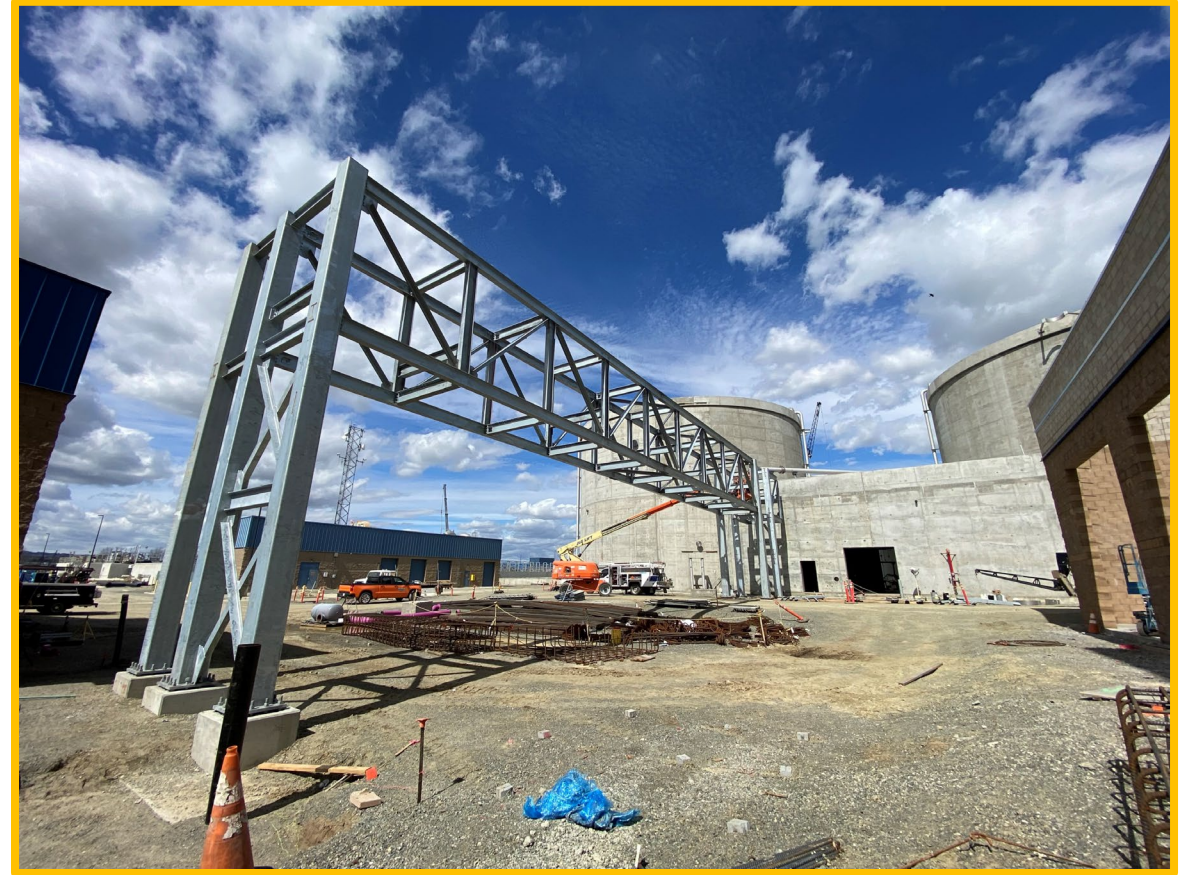
Gas Phase Digester Pipe Bridge
