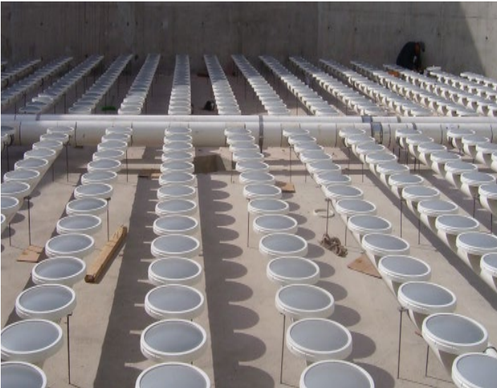
Disc diffuser installation RP-4
