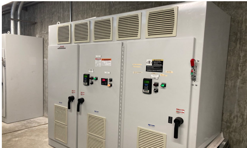
Variable Frequency Drive (VFD)
