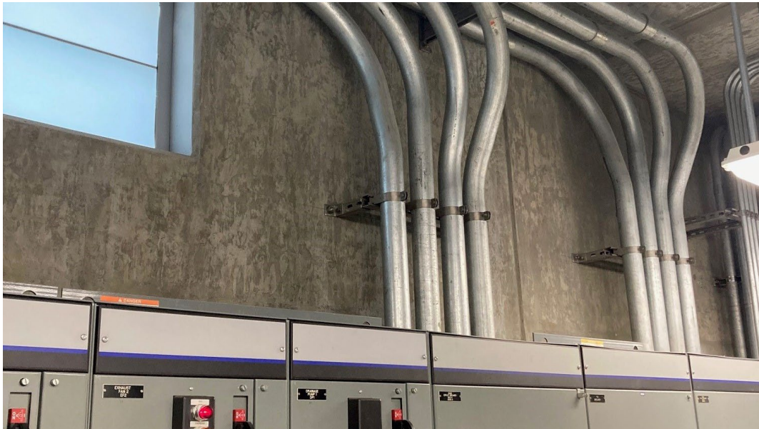
Conduit entering a Motor Control Center (MCC)
