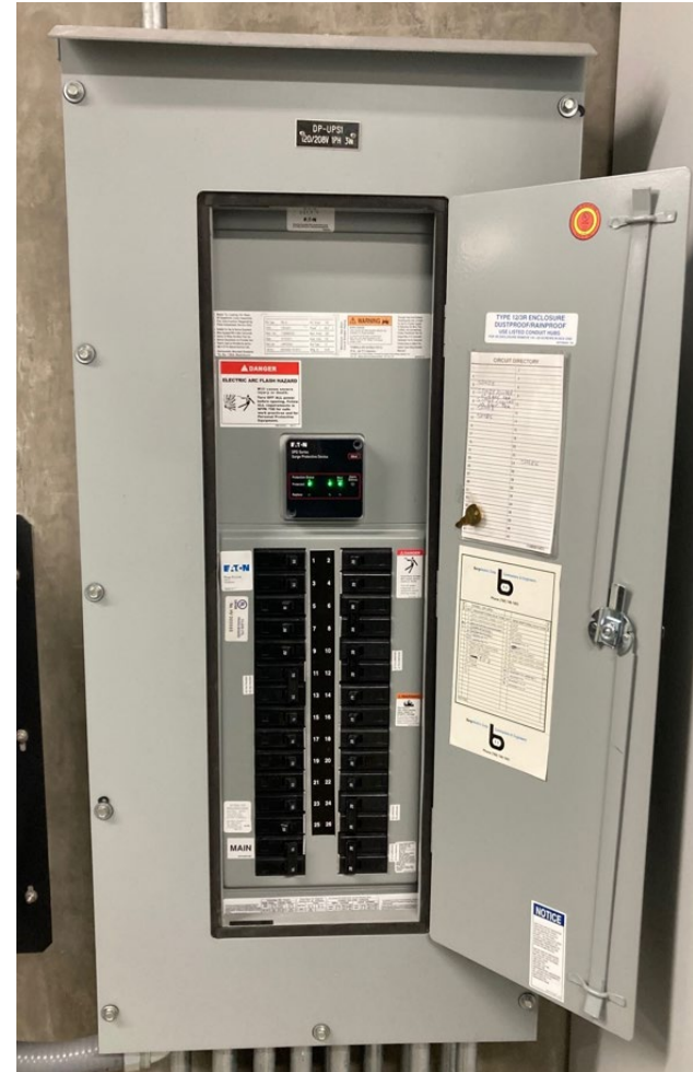
Electrical Breaker Panel
