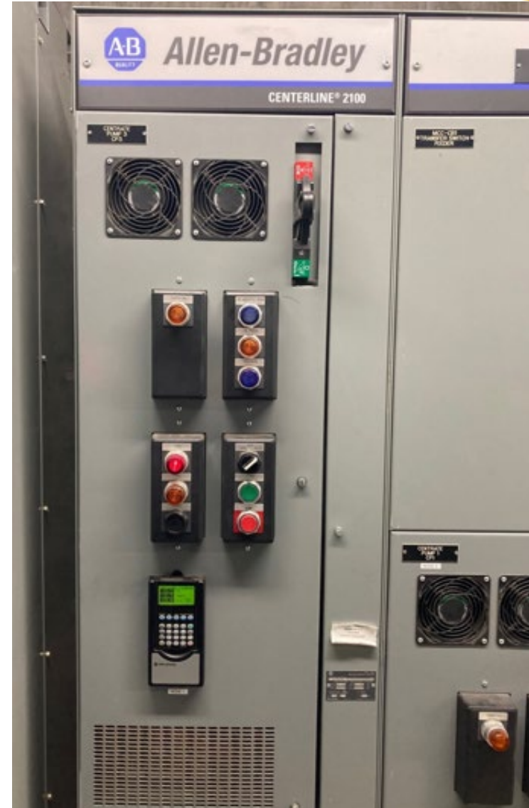
Motor Control Center (MCC)
