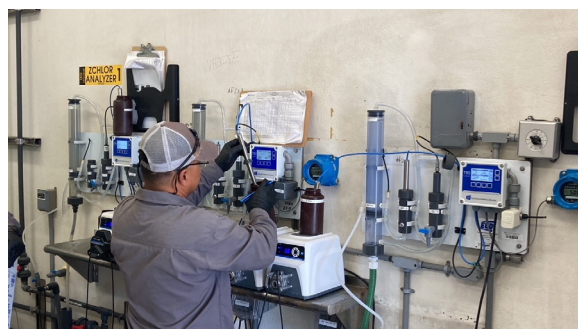
Top Left: RP-1 Polymer Pump Repair Bottom Left: RP-1 Z- Chlorine Calibration
