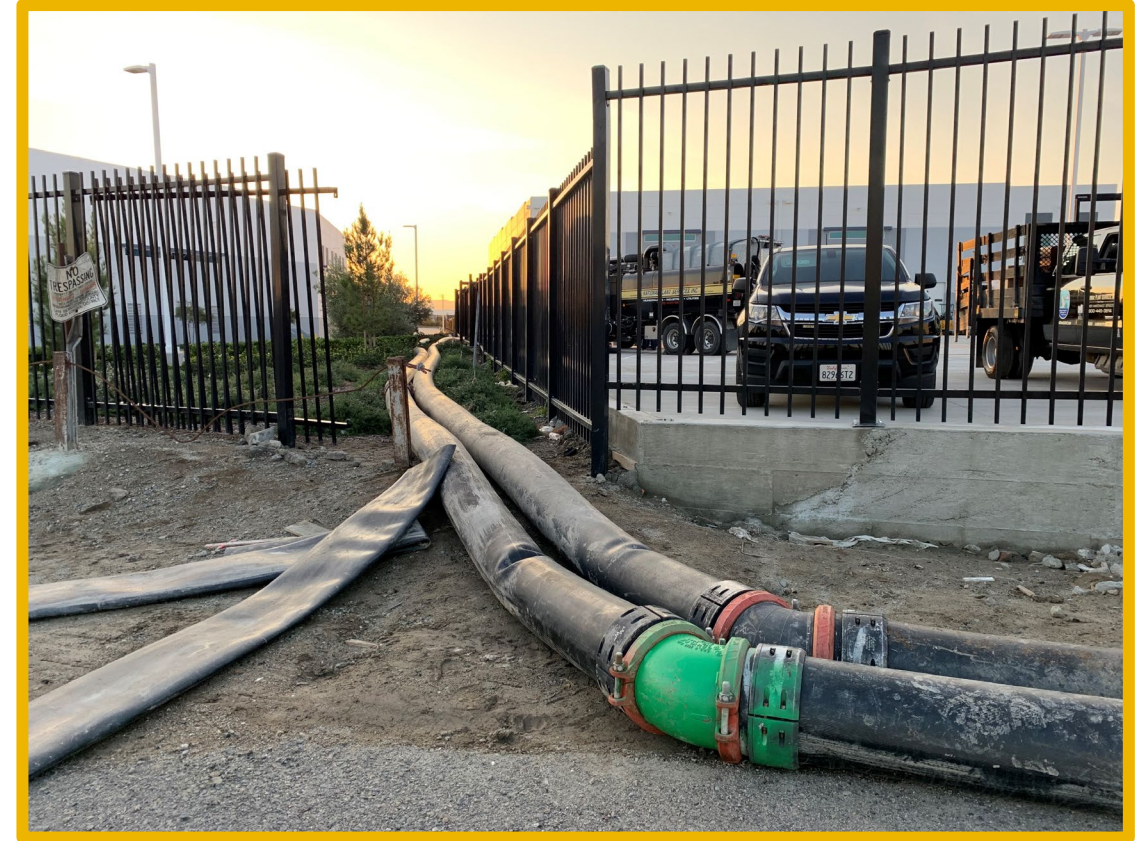
Sewer Bypass - Above Grade Piping
