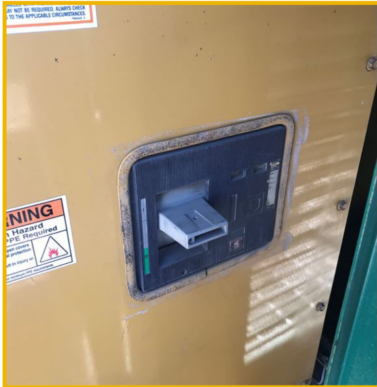
Tripped RP-4 Generator Breaker
