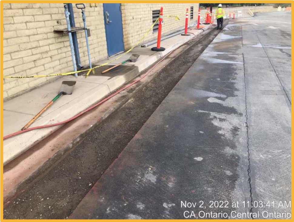
New duct bank north of control building.
