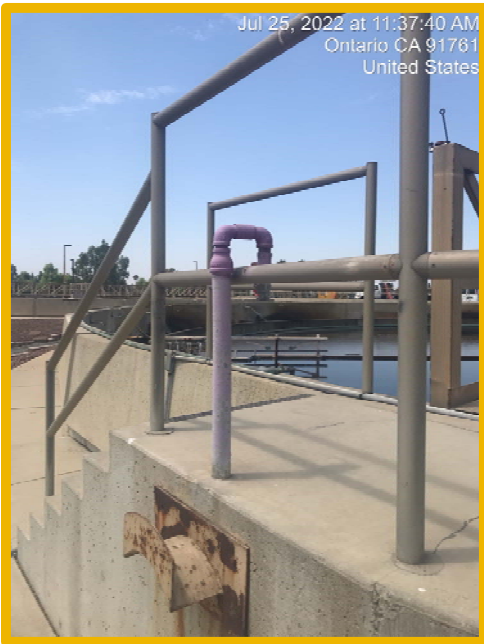
Existing aeration basin sprayers (left) and secondary clarifier hose bibbs (right).
