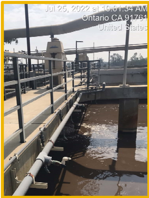
Existing aeration basin sprayers (left) and secondary clarifier hose bibbs (right).
