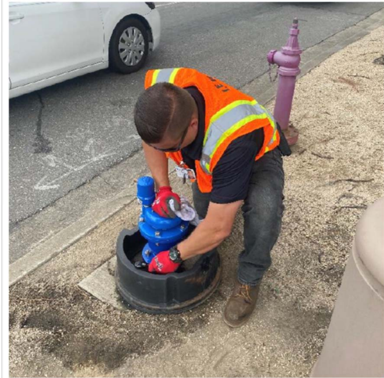
Air & Vacuum Relief Valve Maintenance
