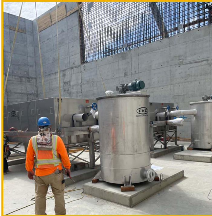
Rotary Drum Thickeners Thickening Building
