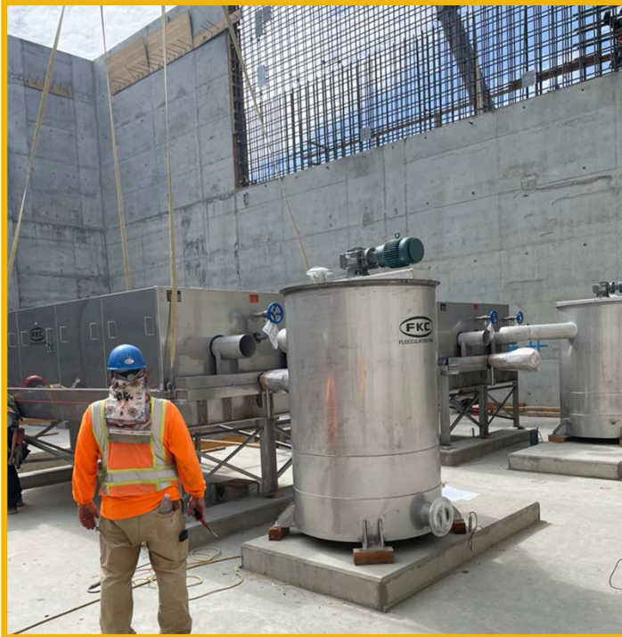
Rotary Drum Thickeners Thickening Building
