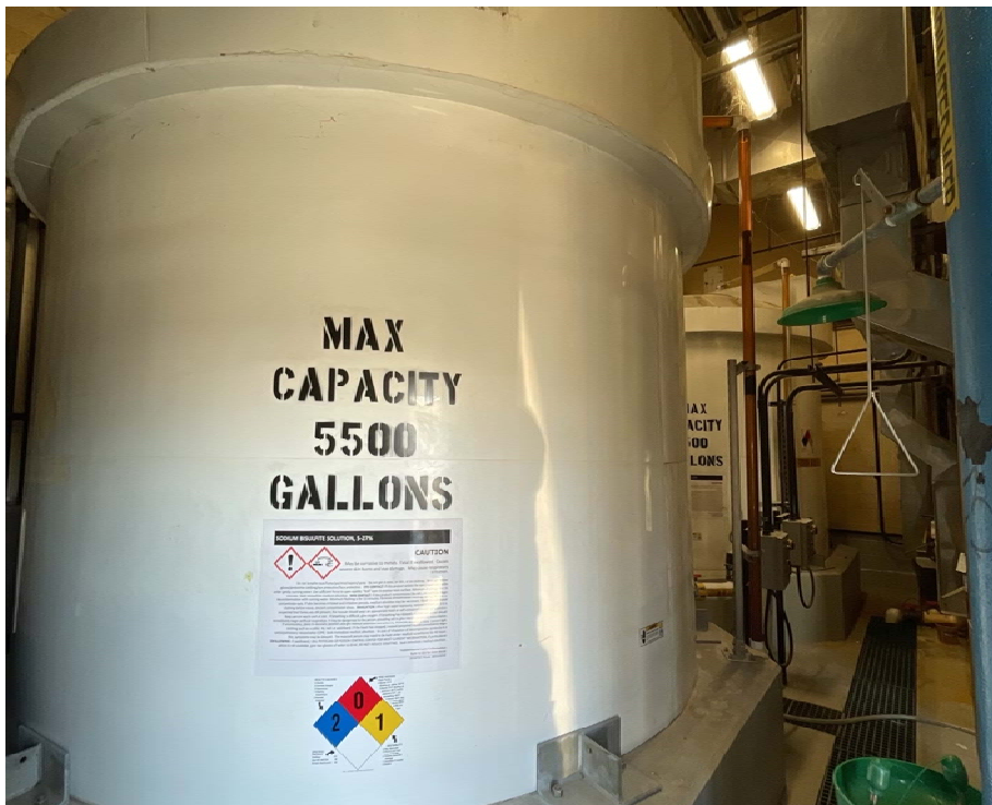
CCWRF SBS Storage Tanks
