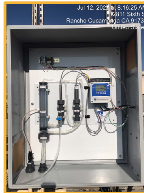
New Free Chlorine Analyzer
