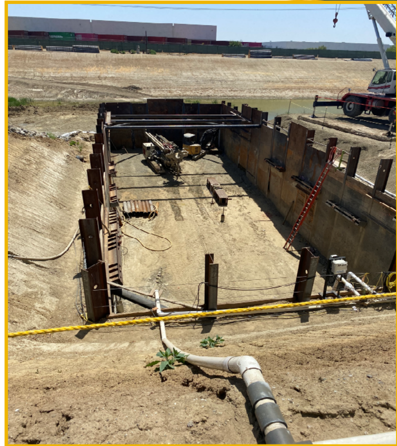
Emergency Overflow Pond Pumps Station
