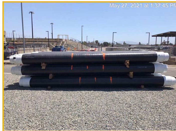
New Hot Water Loop Pipeline
