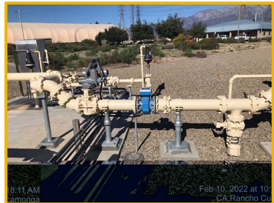
Primary Sludge Wasting
