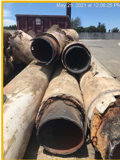
Removed Corroded Line
