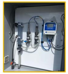
ECD Chlorine Analyzer RP-1
