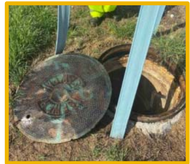
Typical Category 1 & 2 Manhole Requiring Retrofit
