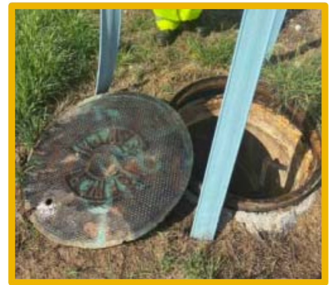
Typical Category 1 & 2 Manhole Requiring Retrofit
