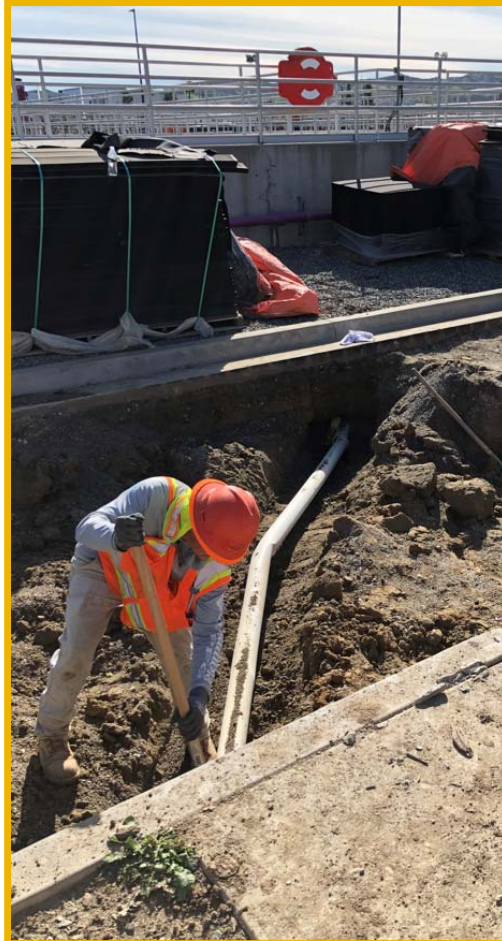
Sodium Hypochlorite Line Break
