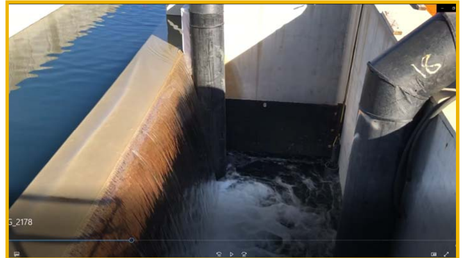
Sodium Hypochlorite Line Break
