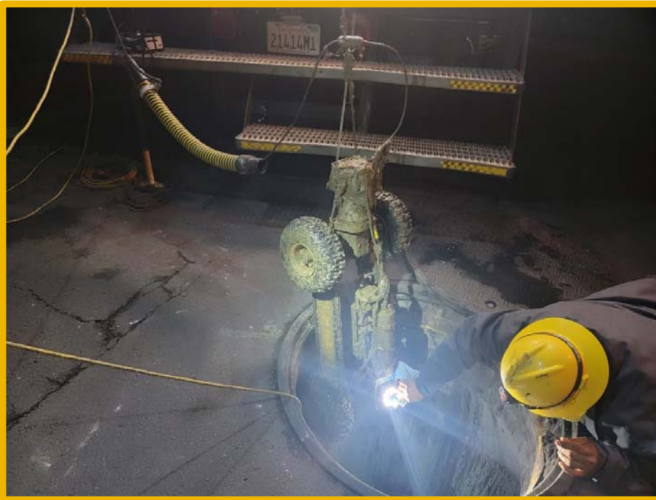
Remote CCTV Entering MH for Inspection
