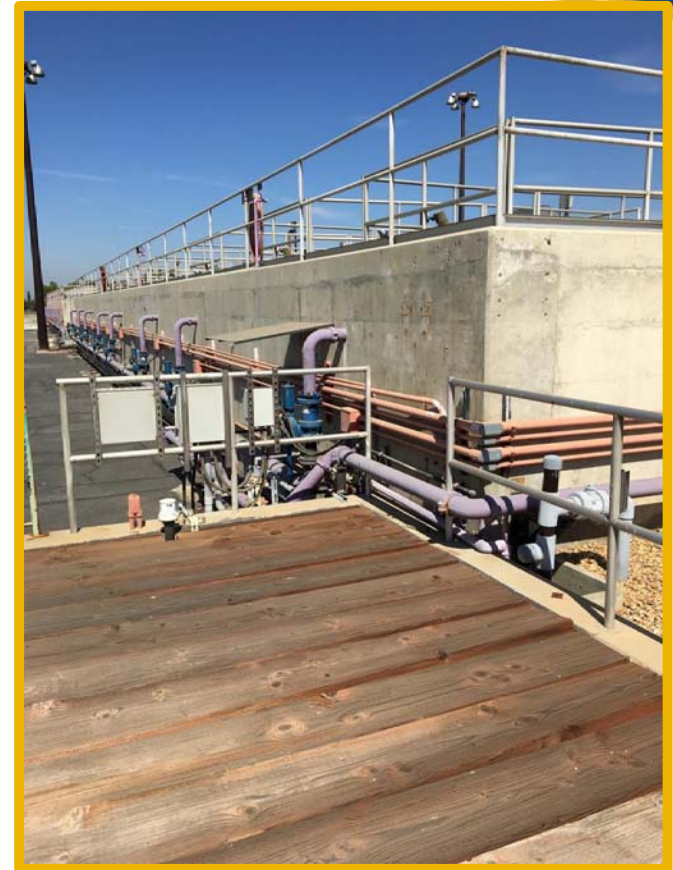
Unsecured Wood Plank Covers
