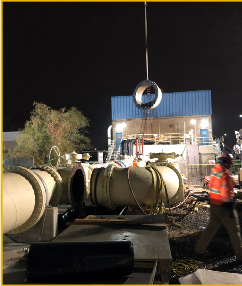
Influent Pump Station Bypass Valve Install
