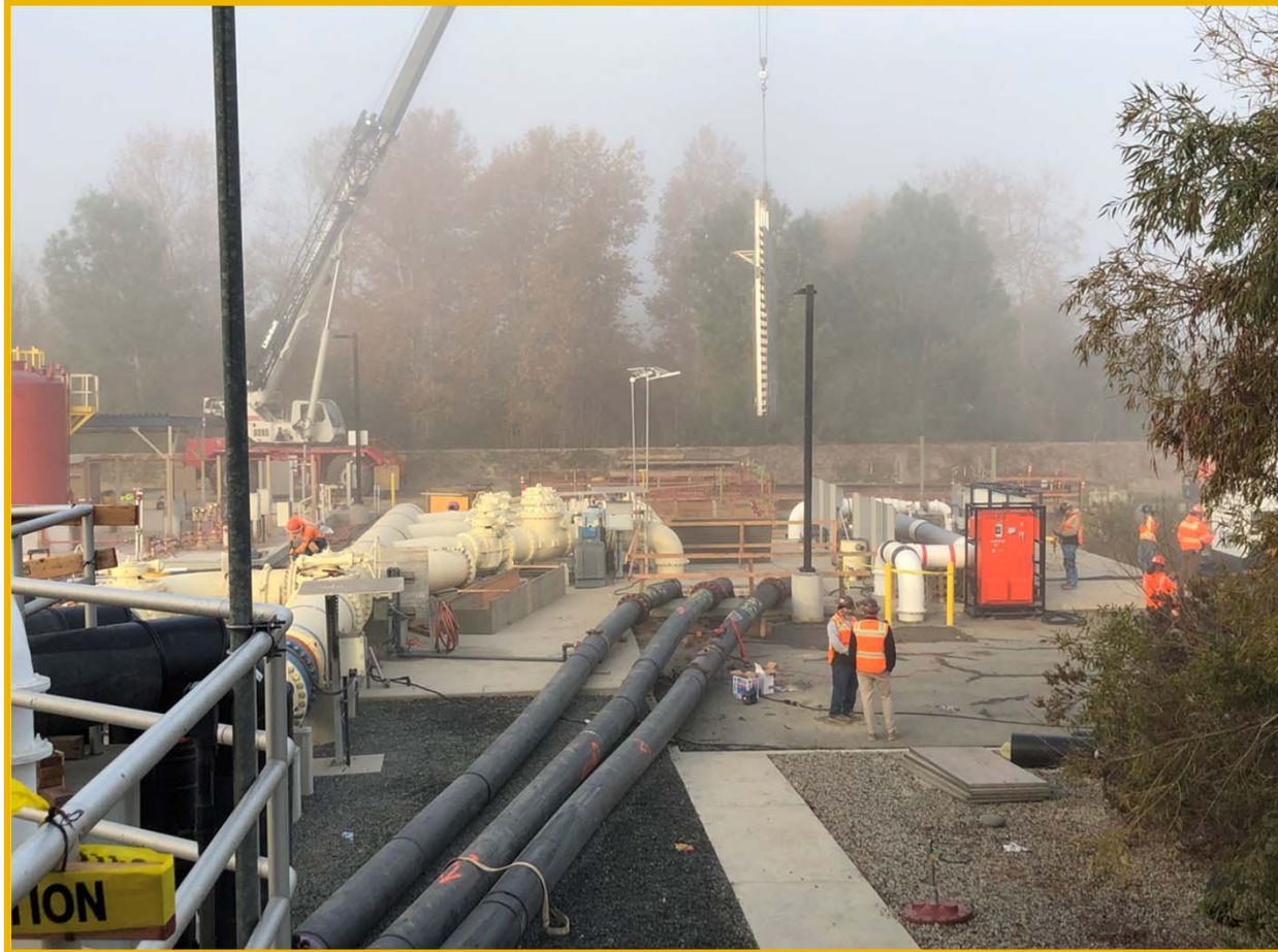
Influent Pump Station Bypass Valve Install
