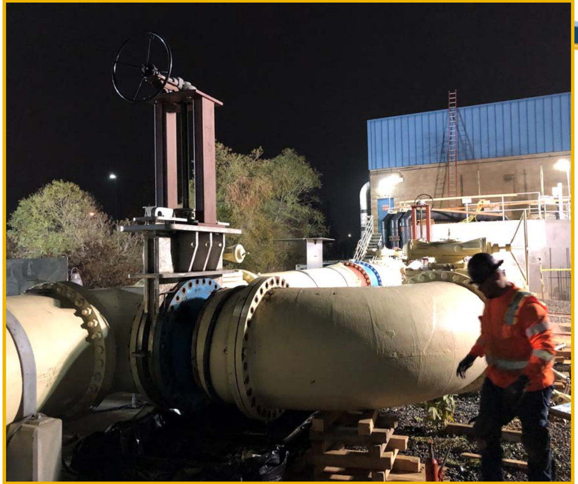
Influent Pump Station Bypass Valve Install
