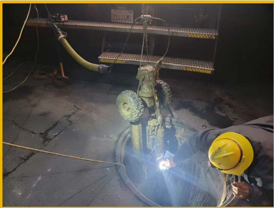
Remote CCTV Entering MH for Inspection
