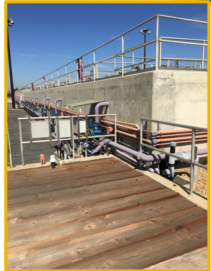
Unsecured Wood Plank Covers
