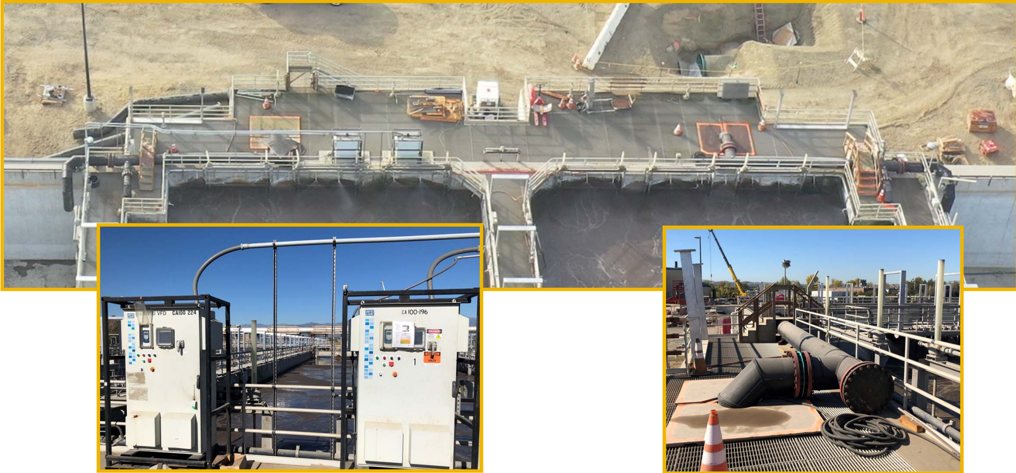
Aeration Basin ( Temporary Mix Liquor Return Pumps)
