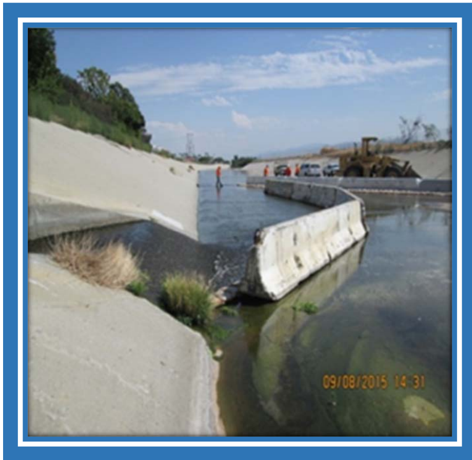
Flow Diversion Set-up
