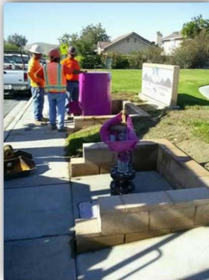
Wineville recycled water pipeline air release valve and blow-off assembly at Chaparral Park in Fontana, CA
