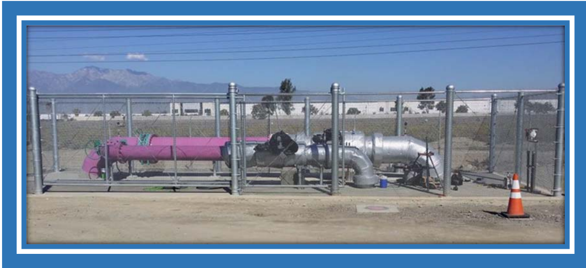
Valve Station at RP-3
