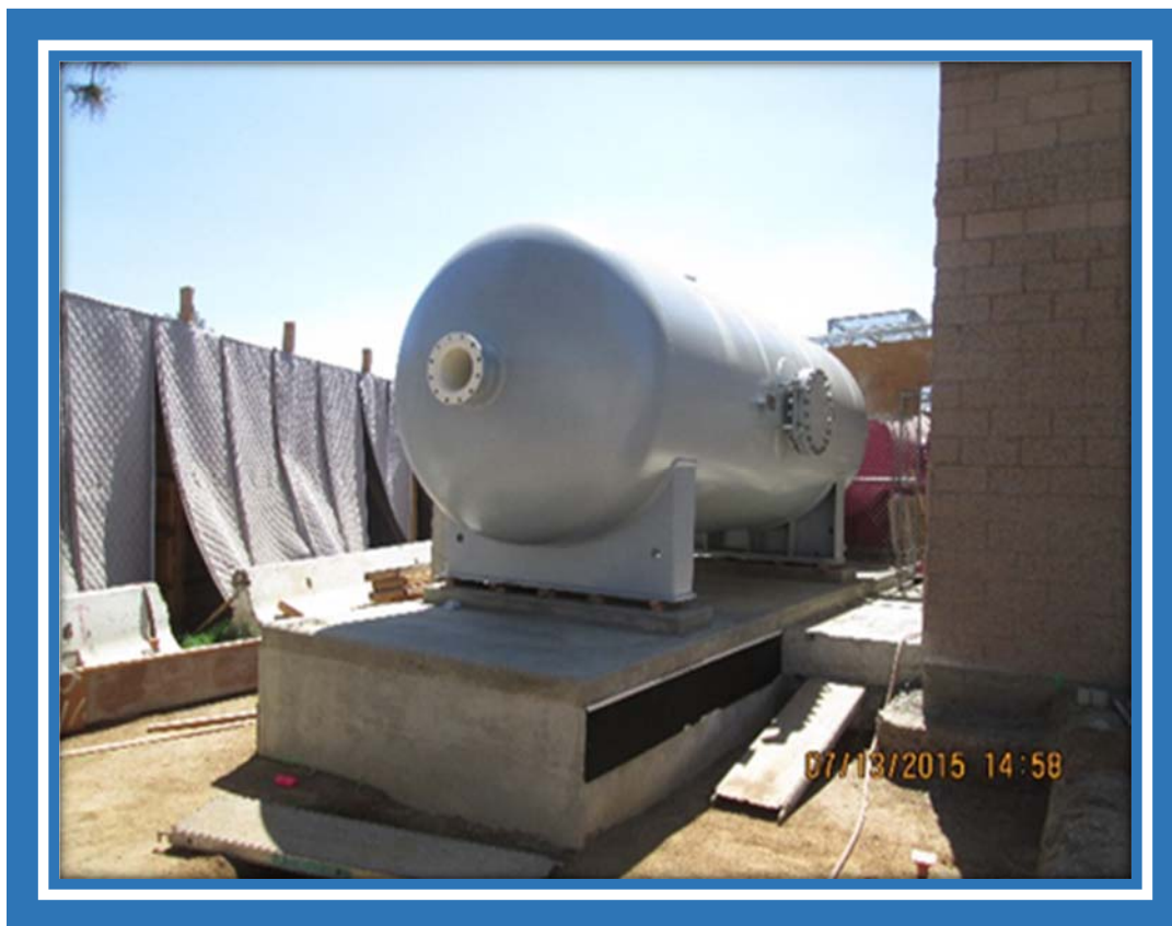
Surge Tank Installed on Pad
