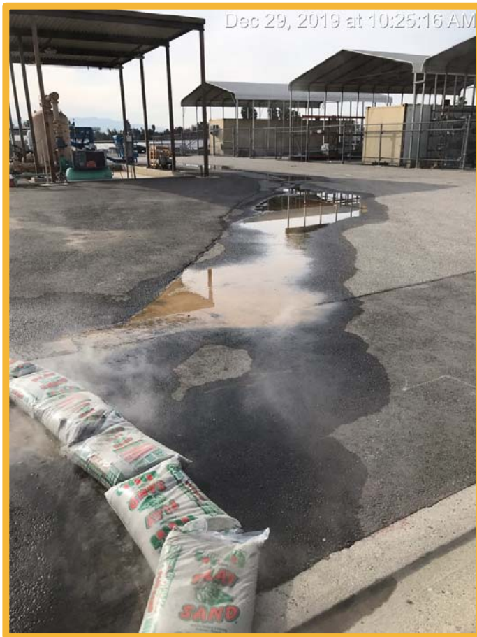
Hot Water Loop Leak
