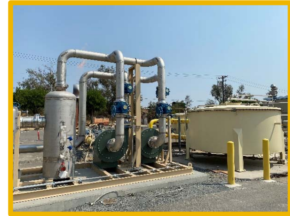
Gas Blower Skid and Foundation
