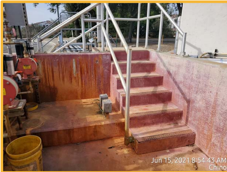
Ferric Chloride Containment
