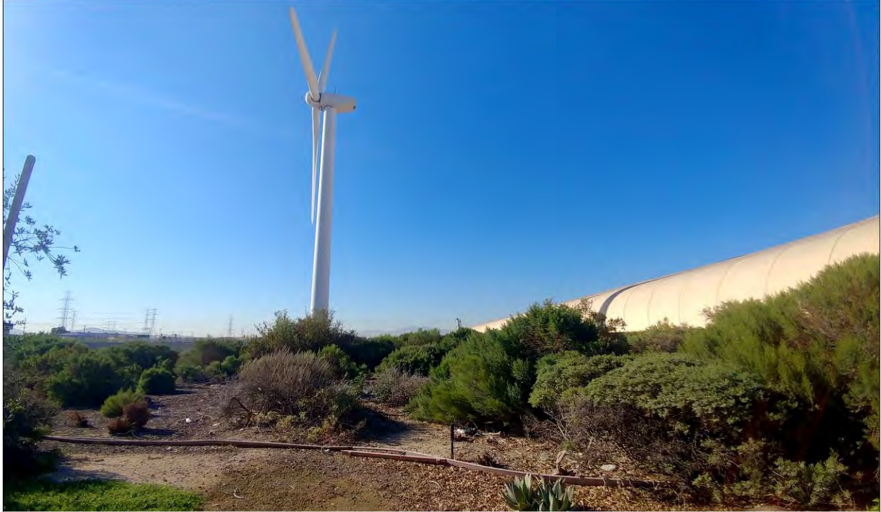
Figure 3. Typical landscape within the project area. (View to the south; photograph taken on September 22, 2021)
