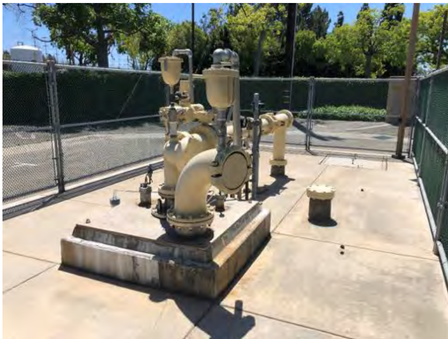
Figure 4-5. Example Injection Well Site
