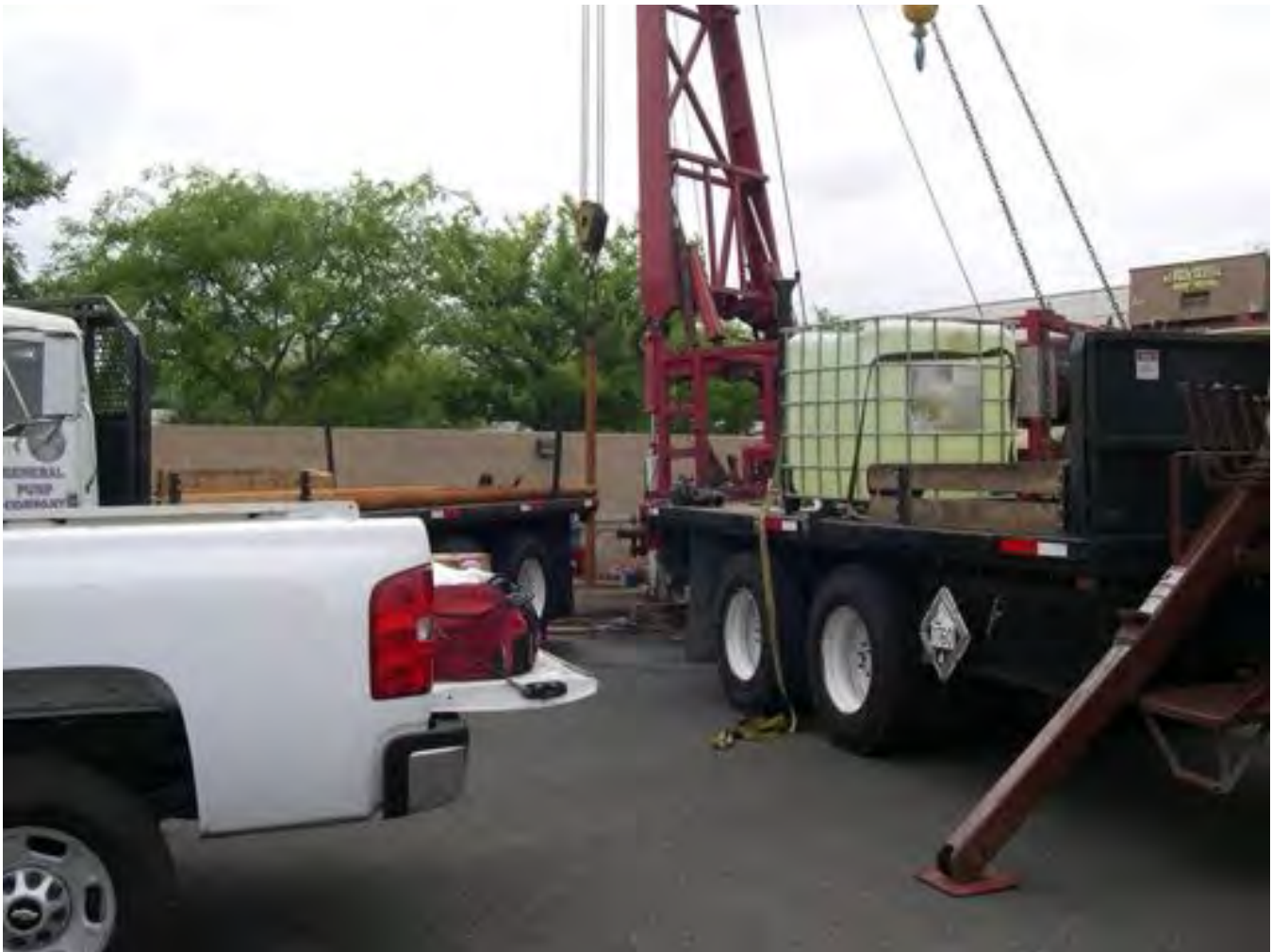
Figure 5-1. Well Rehabilitation Activities
