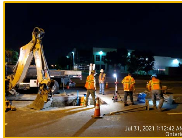
Excavating the Valve on Ontario Mills Parkway
