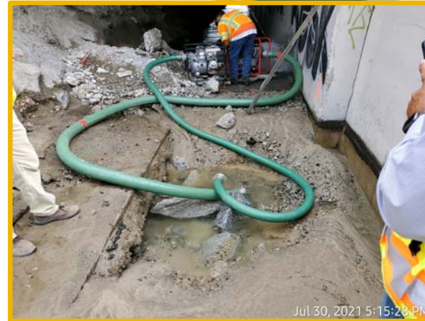
Dewatering 42-inch Effluent Pipeline
