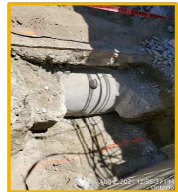
42" Pipeline Leak Repaired
