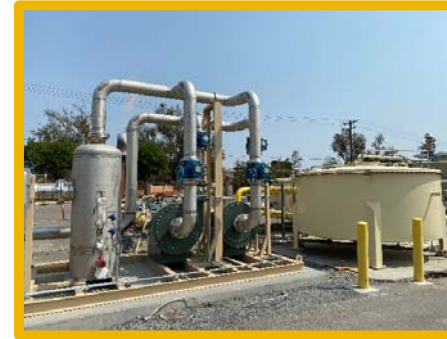
Gas Blower Skid and Foundation
