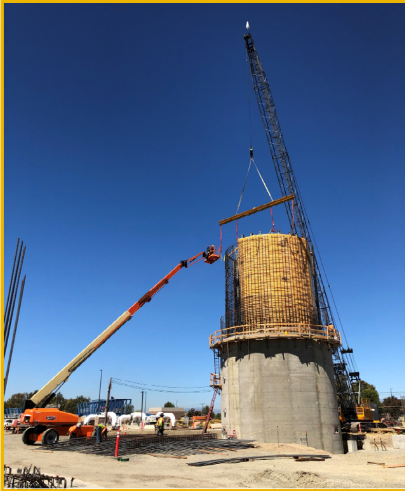
Acid Phase Digester – 2 nd Lift of Walls
