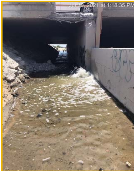
Leaking 42-inch Pipeline
