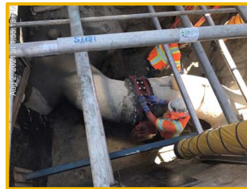
South Isolation Valve Bypass
