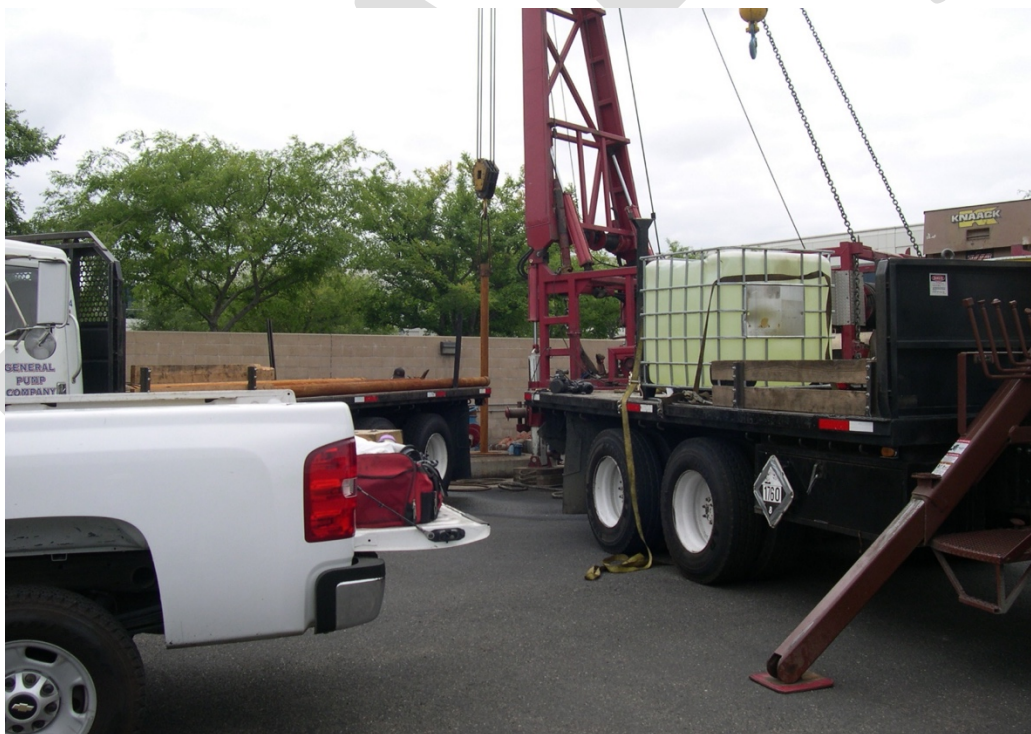
Photo 2: Well Rehabilitation Activities
