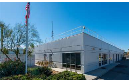
Chino Basin 1 Desalter
