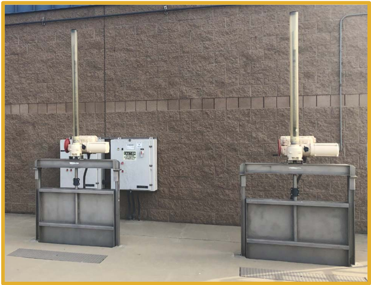
RP-5 BAR SCREEN INLET & OUTLET GATE ACTUATORS REPLACEMENT TO EXTEND ASSET LIFE
