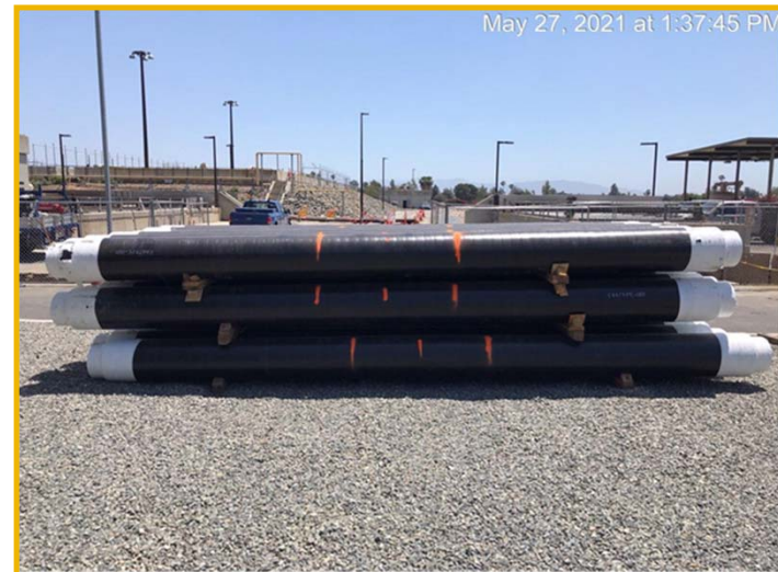
New Hot Water Loop Pipeline
