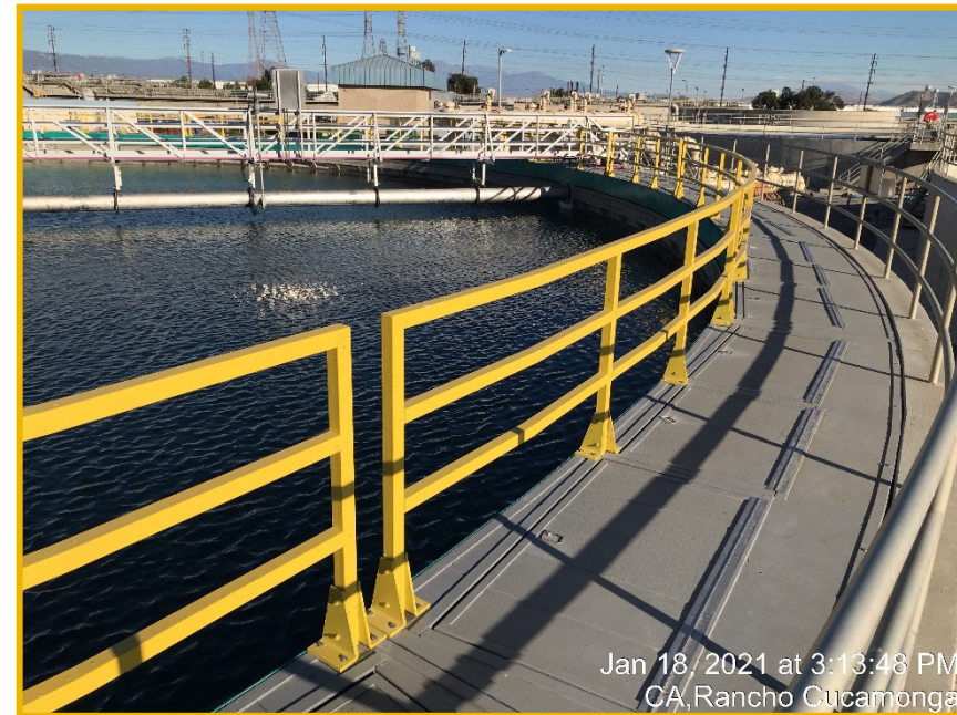
New RP-4 Secondary Clarifier Channel Covers
