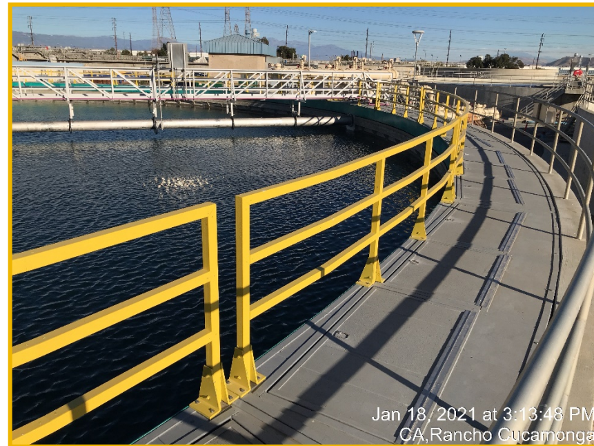
New RP-4 Secondary Clarifier Channel Covers
