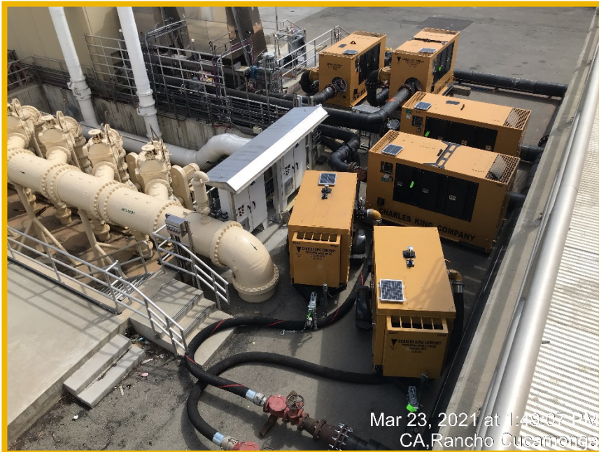
RP-4 Headworks Bypass in Progress
