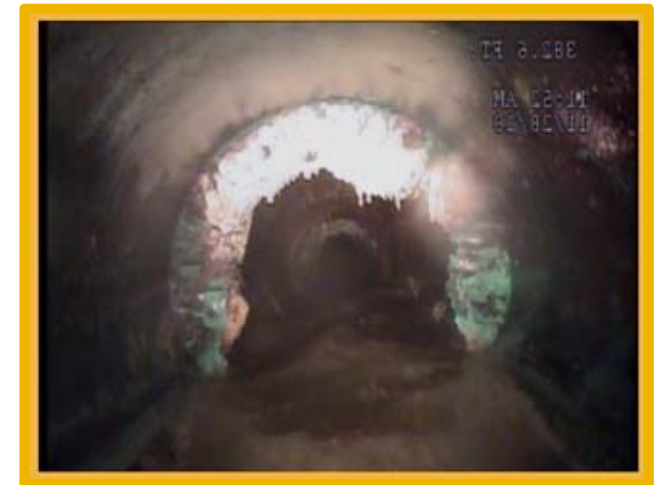
Trunk Sewer Coating Failure
