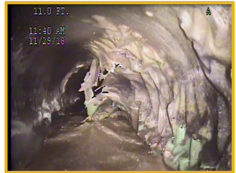
Trunk Sewer Coating Failure
