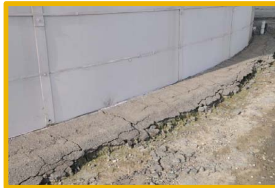
Bottom Plate Extension Covered in Asphalt
