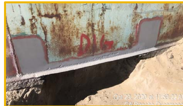
Good Bottom Plate Extension Condition
