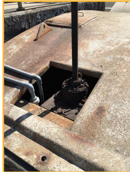
Partial Old Effluent Structure View
