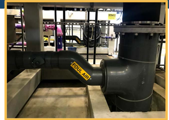
Existing Foul Air Line Connection
