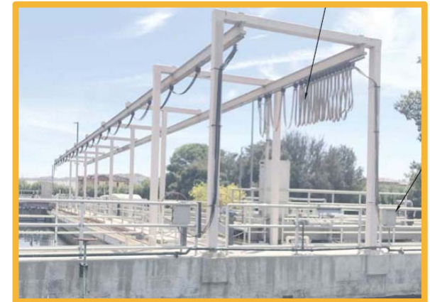
Existing Cables for Traveling Bridge
