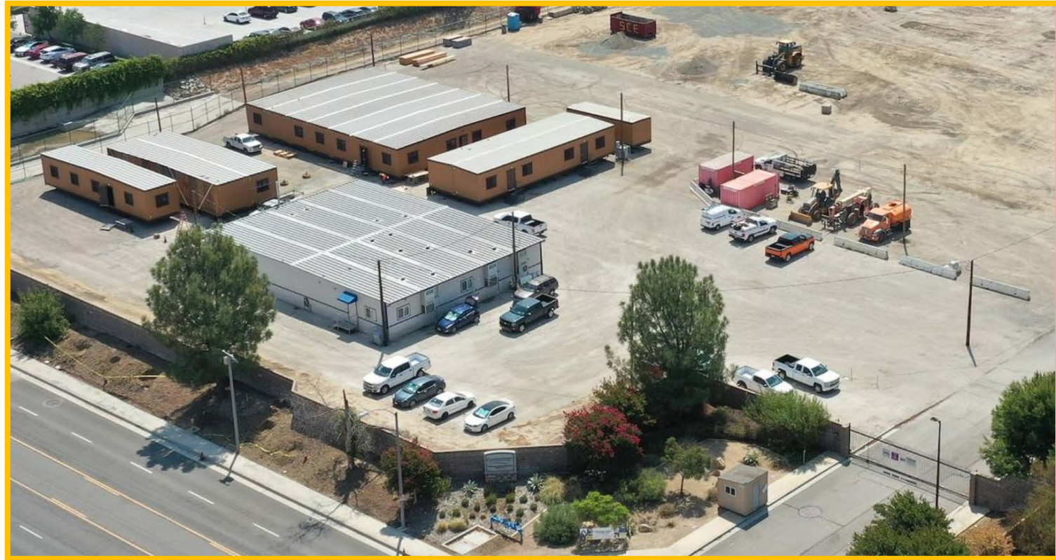
Trailer Complex Mobilization
