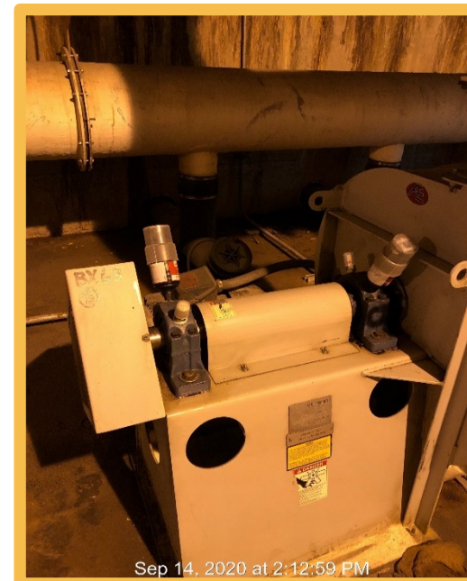
Sensor Installed at IERCF
