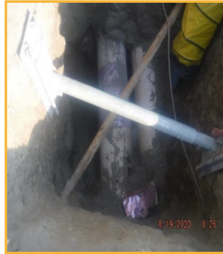
Existing Dual Pipelines
