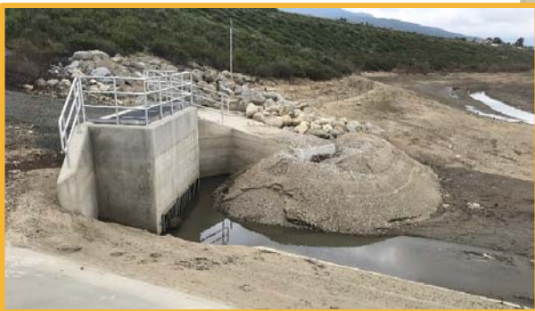
Alluvial deposits near new inlet structure
