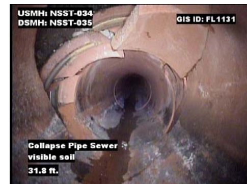
NRW North System South Trunk Pipe – Identified Damage Several Years Ago
